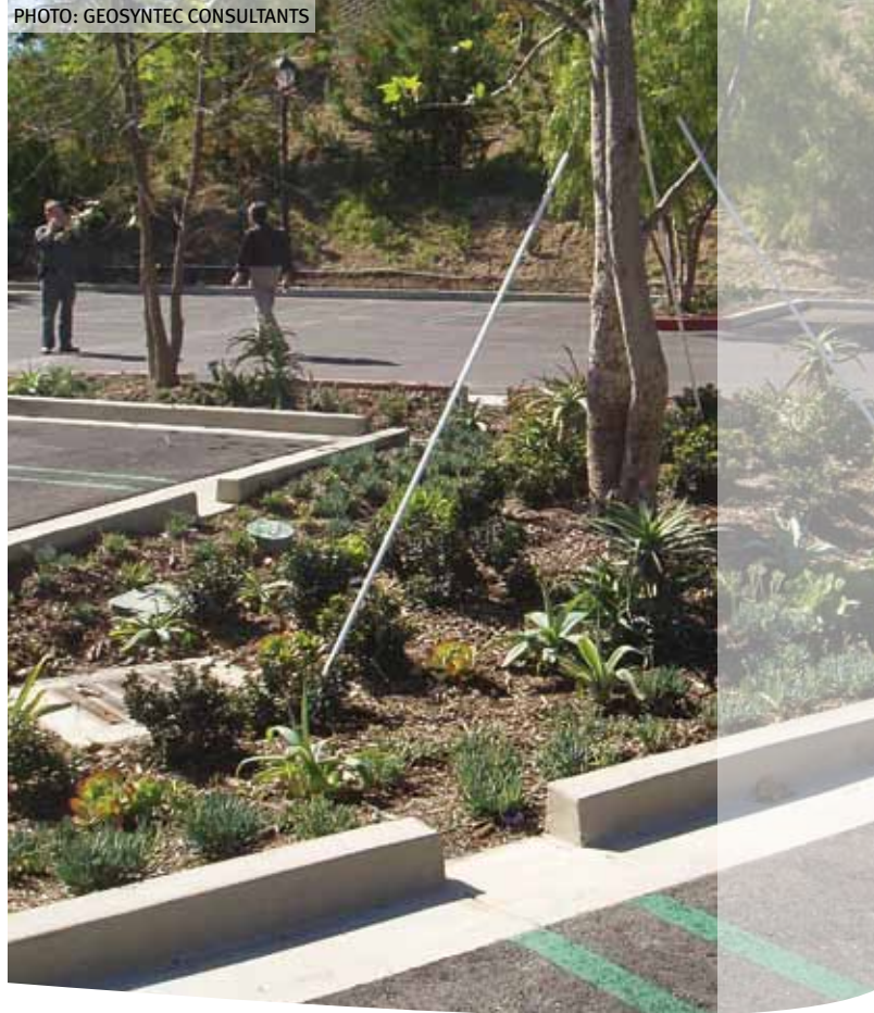
Figure 4. Example of On-site LID BMP in Parking Lot
