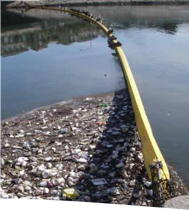
Trash Boom between the Lincoln Blvd and Culver Blvd Overpasses in Ballona Creek
