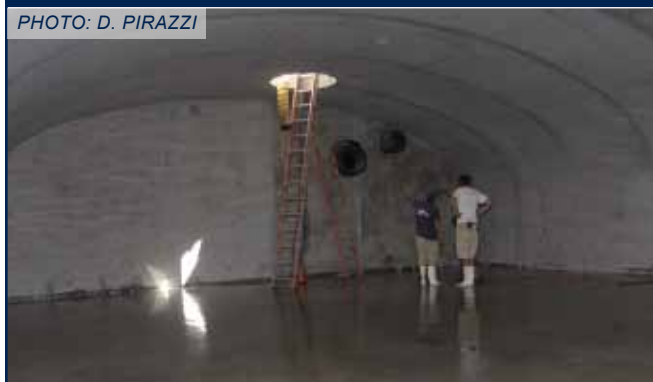
Figure 6. Inside the Low Flow Diversion Vault
