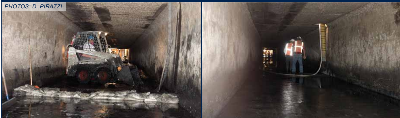
Figure 7. 1,000-Foot Culvert: During and Post-Cleaning
