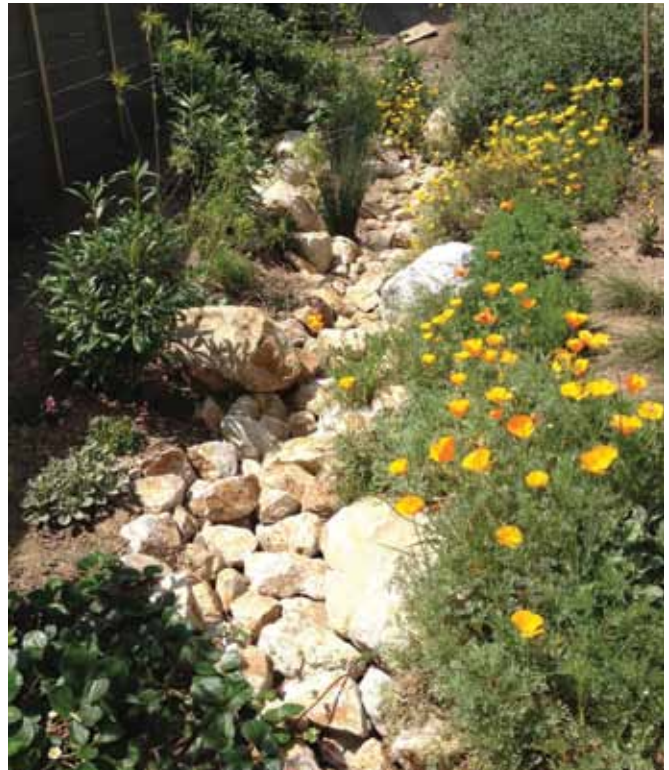
FIG. 8B. Rain garden under construction after a big rain event with some preliminary landscaping.
