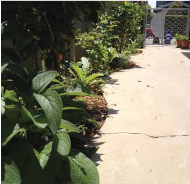
FIG. 7. The original driveway was retained for bike riding and skating but 4' of it was removed for better infiltration and to plant the fruit trees and perennials.
