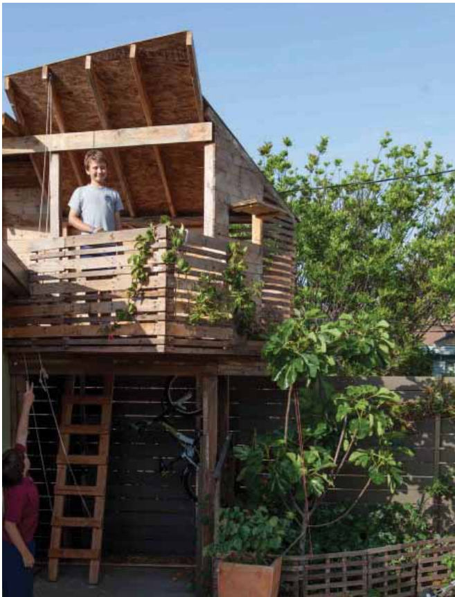
FIG. 17. A tree house made with recycled wood lath and pallets, next to a young fig tree and the berry patch.
