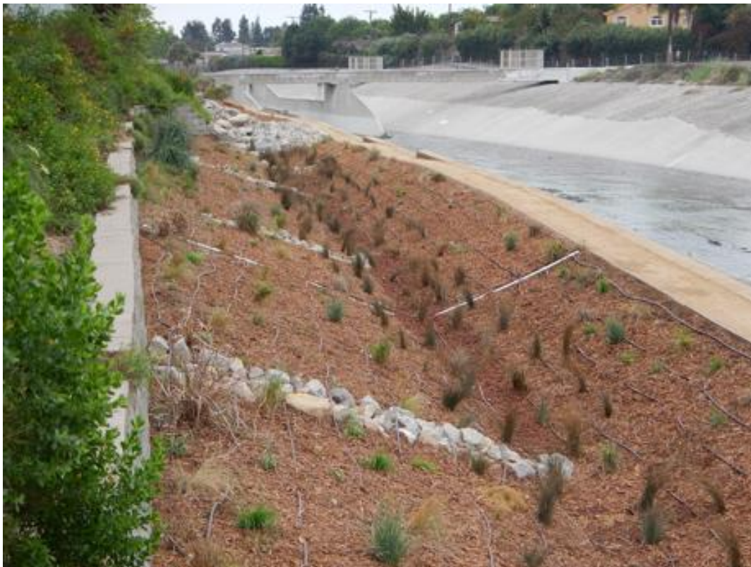
Figure 1.2.1-3. The newly planted Culver City rain garden located along the Ballona Creek. This 1000-ft rain garden intercepts runoff from commercial buildings and parking lots located along Jefferson Blvd. Photo: Ivan Medel, The Bay Foundation
