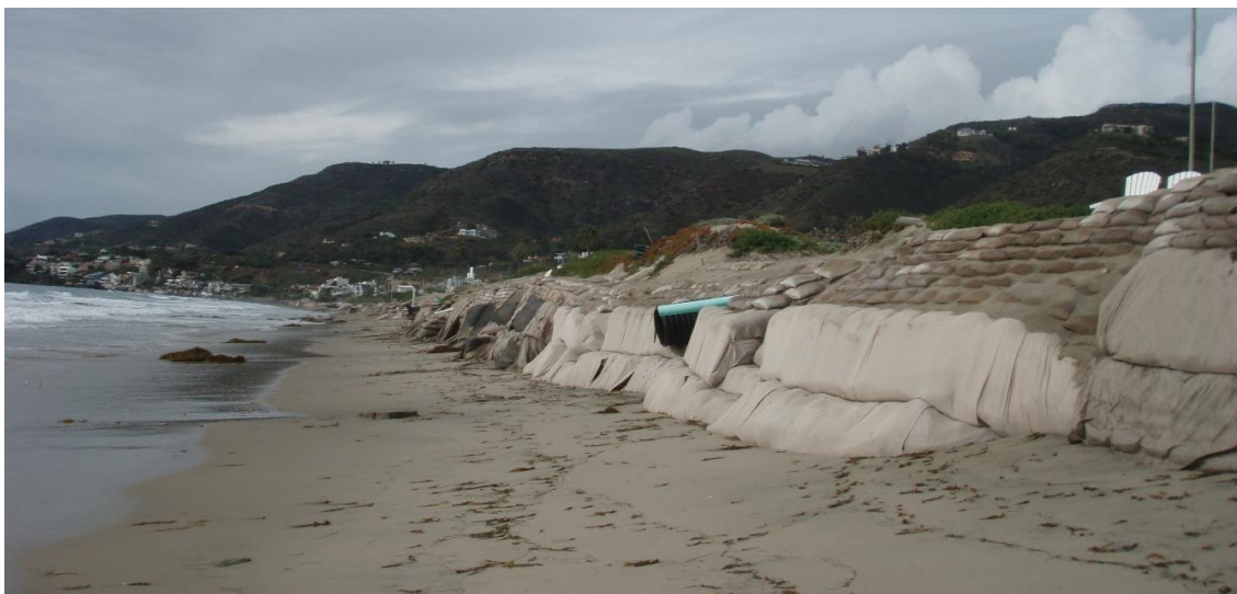
Figure 4.2-2. Sandbags protecting property and contributing to beach erosion on Broad Beach, circa 2008. Photo Credit: Lia Protopapadakis, The Bay Foundation
